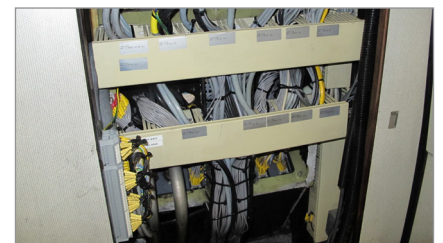
▲ Top photo: before preventive maintenance. Bottom photo: after preventive maintenance.
